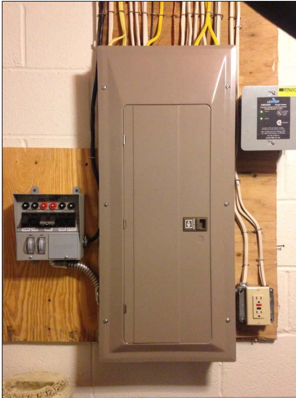
Figure 13 - Here's the transfer switch (gray box on left) wired to the home's electrical panel. The black cable exiting the right of the transfer switch runs to the socket in the garage.
