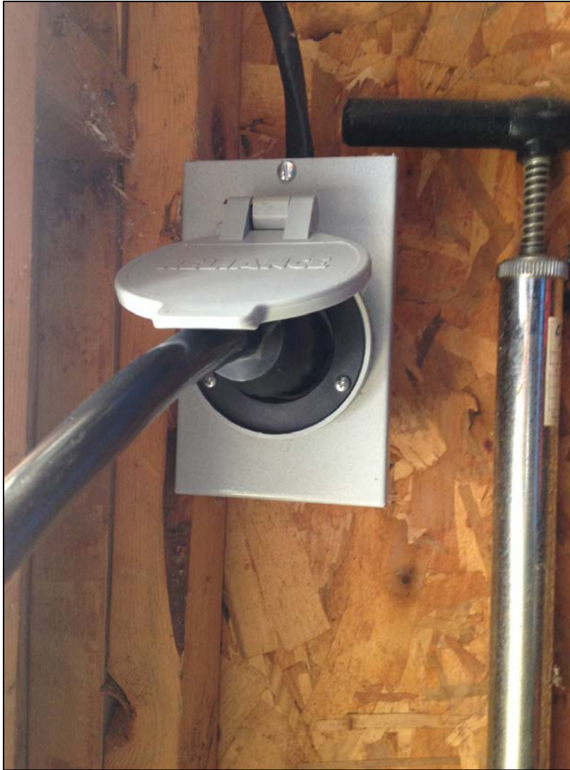
Figure 12 - The socket in the garage for connecting the inverter to the transfer switch.
